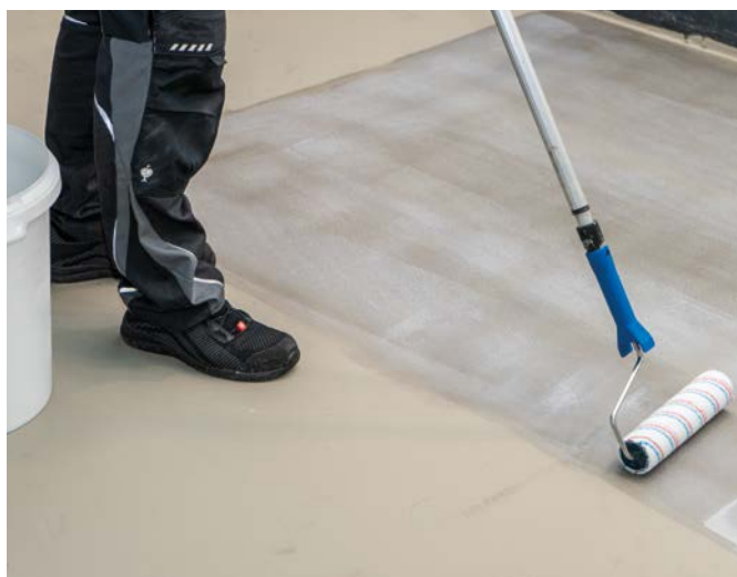
Apply a suitable tackifier
