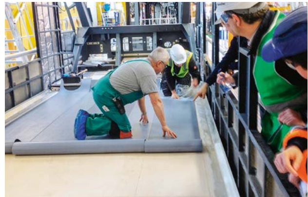
Ongoing nora® nTx installation
